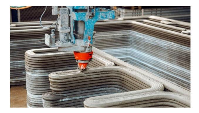
A COBOD BOD2 3D construction printer builds structural elements of a Houston home that will be the first multistory 3D-printed structure in the United States. Credit: Leslie Lok and Sasa Zivkovic
