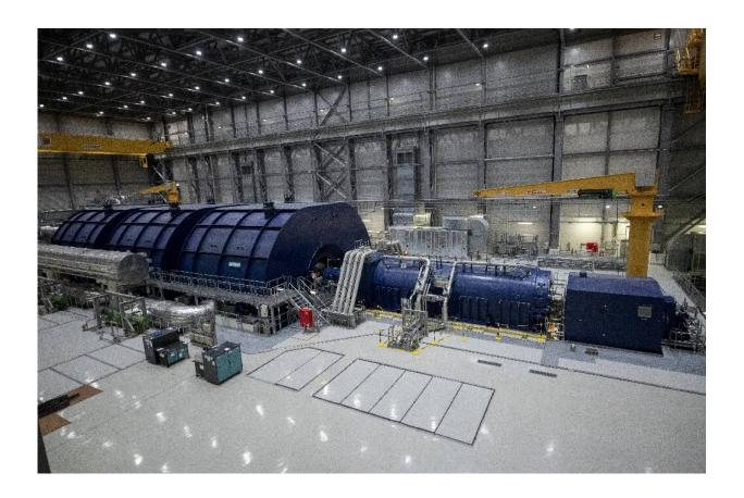
The almost 300-degree Celsius (572 F) steam gushing from the reactor turns the over 60-meter-long turbine up to 25 times every second.
