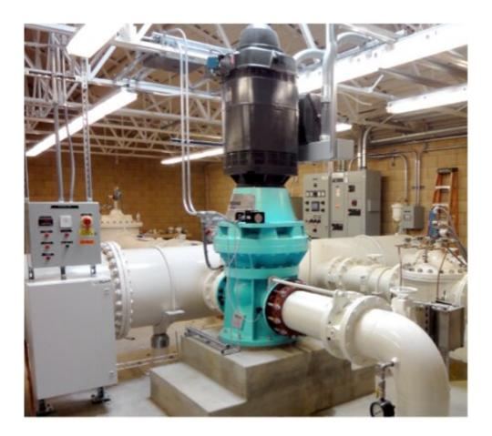
A hydropower turbine is installed into an existing drinking water distribution system in Palmdale, California. Credit: Canyon Hydro
