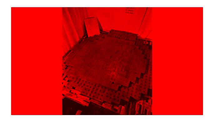
Scientists built Chicago Pile 1, the world's first nuclear reactor, layer by layer beneath the University of Chicago's Stagg Field. In this photo, the layer shows graphite bricks with small holes for uranium or control rods used during the experiment. Credit: Argonne National Laboratory.
