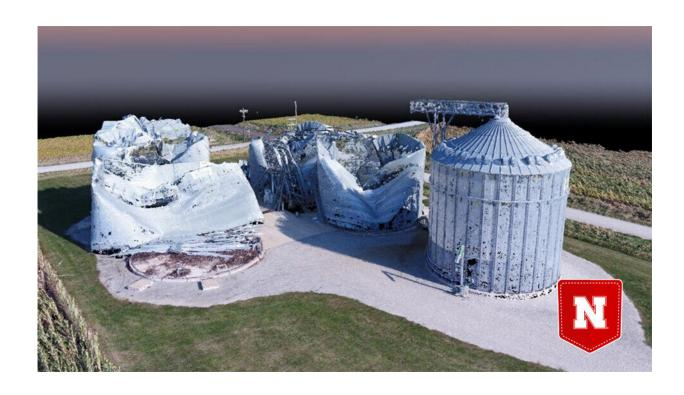
A 3D rendering of grain bins following an August 2020 windstorm. The rendering was produced with the aid of lidar—near-infrared laser beams fired at the structures by a drone flying above the site. Credit: University of Nebraska-Lincoln
