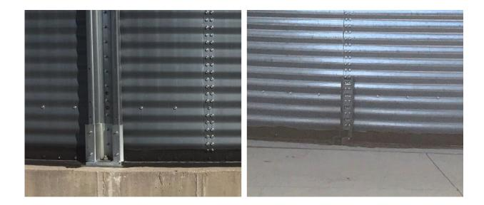
A vertical stiffener on a commercial bin (left), as compared with an anchorage clip found on a typical farm bin (right). Credit: Christine Wittich
