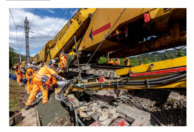
Track-work machines are noisy and emission-intensive and expensive to operate and maintain. The special machines carry out several work steps simultaneously, for example renewing the track or grinding rails. Credit: Lunghammer—TU Graz
