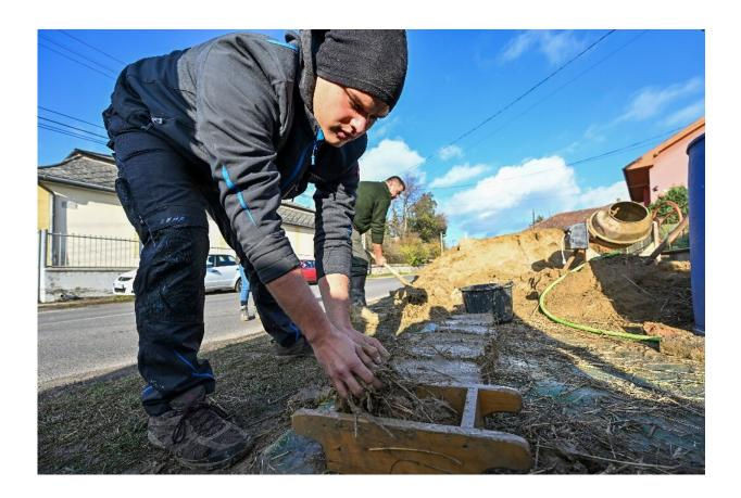
Rammed earth construction, dates back to Neolithic times but is seeing a revival thanks to its tiny ecological footprint and energy efficiency.
