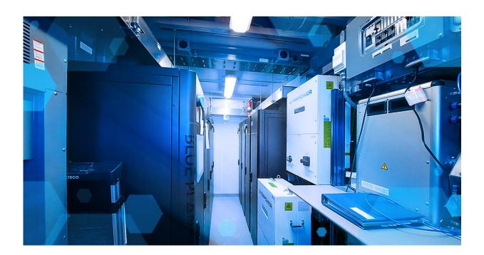
INL's Microgrid in a Box includes 320 kilowatt-hours of battery storage, and can tie seamlessly into a modern electrical grid and coordinate the distribution of electricity for a small village, military base or other critical infrastructure building. Credit: Idaho National Laboratory
