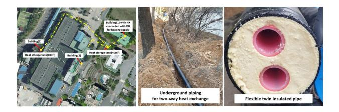
Photo of heat piping network. Credit: Korea Institute of Civil Engineering and Building Technology
