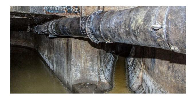
Beneath the Bahnhofstrasse in Zurich, a sewer conveys wastewater to the treatment plant. Rainwater is channelled through a separate pipe. Credit: Max Maurer / ETH Zurich
