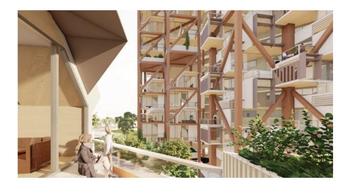
New structures providing communal spaces could be built from the ground up, providing additional bracing to the existing towers rather than adding any load to them. Credit: George Avraam
