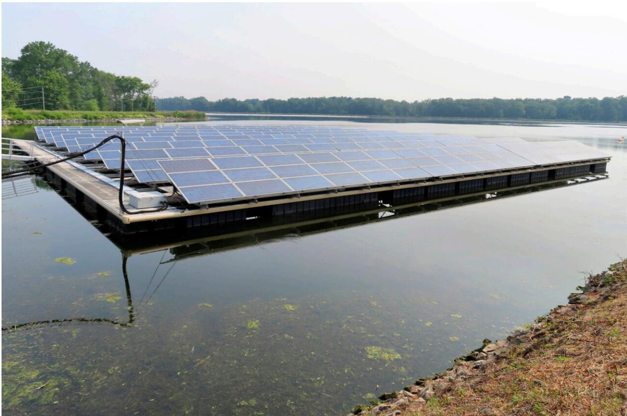
Solar panels from a smaller pilot project are shown, Tuesday, June 6, 2023, a water treatment plant in Millburn, N.J., where a larger array of floating solar panels provides enough electricity to power 95% of the treatment facilities electrical needs. Credit: AP Photo/Wayne Parry
