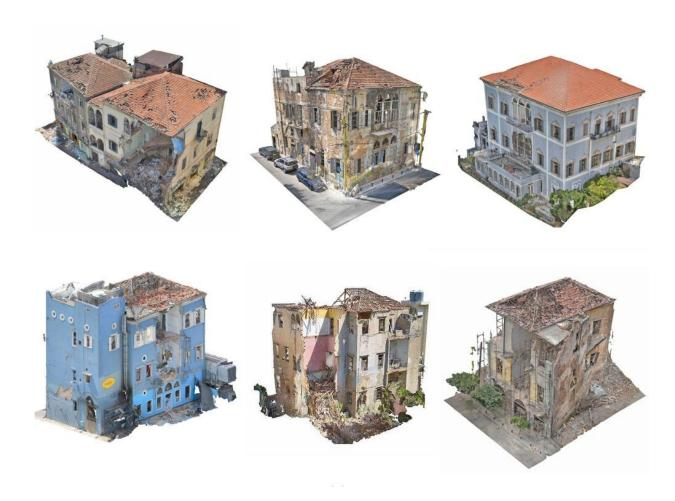
The researchers documented damaged buildings in Beirut and used the images to generate 3D models detailing their structural deformations. Credit: Joe Kallas/Penn State
