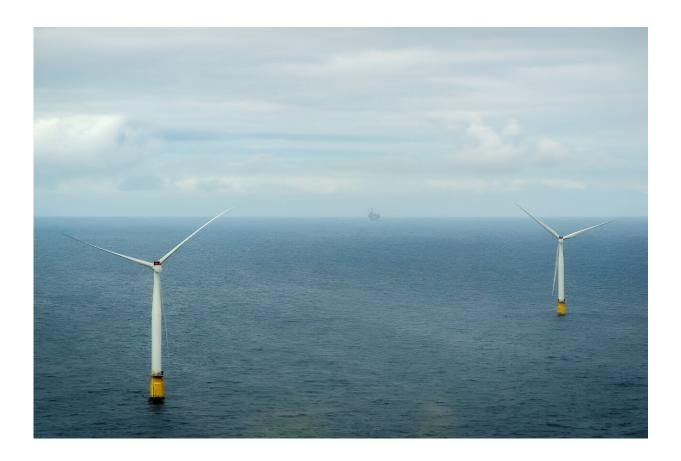
The turbines of Hywind Tampen wind farm are built on floating platforms that are anchored to the seabed.
