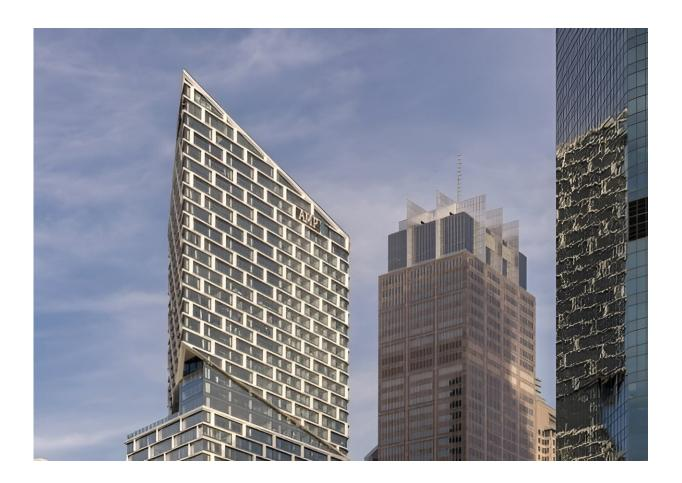
By upcycling and expanding the AMP Tower to create Quay Quarter Tower, rather than doing a knock-down rebuild, architecture firm 3VN saved 7,500 tons of  $CO_2$ . Credit: Adam Monk
