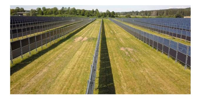
Placing vertical solar panels on farming land allows for energy production and higher yields. Credit: (Wikimedia Commons), CC BY-NC-SA
