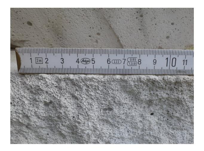
Air is inserted into Raac during construction, making it a light-weight material. Credit: <u>Wikimedia</u>, <u>CC BY-SA</u>
