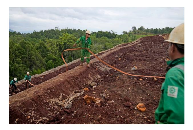
Workers prepare to to carry out hydroseeding to plant grass seed on a slope at PT Vale Indonesia's nickel mine in Sorowako, South Sulawesi, Indonesia, Tuesday, Sept. 12, 2023. As demand for materials needed for batteries, solar panels and other components vital for cutting global emissions rises, carbon emissions by miners and refiners will likewise rise unless companies actively work to decarbonize. Credit: AP Photo/Dita Alangkara
