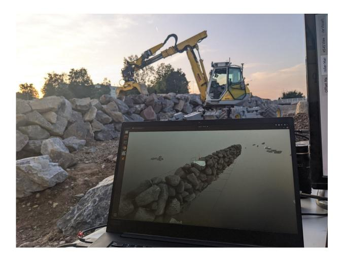
Computational planning and stone placement using the autonomous excavator HEAP, Circularity Park in Oberglatt, Eberhard AG, 2021–2022. Credit: Gramazio Kohler Research, ETH Zurich, Eberhard AG. Photo: Ryan Luke Johns.
