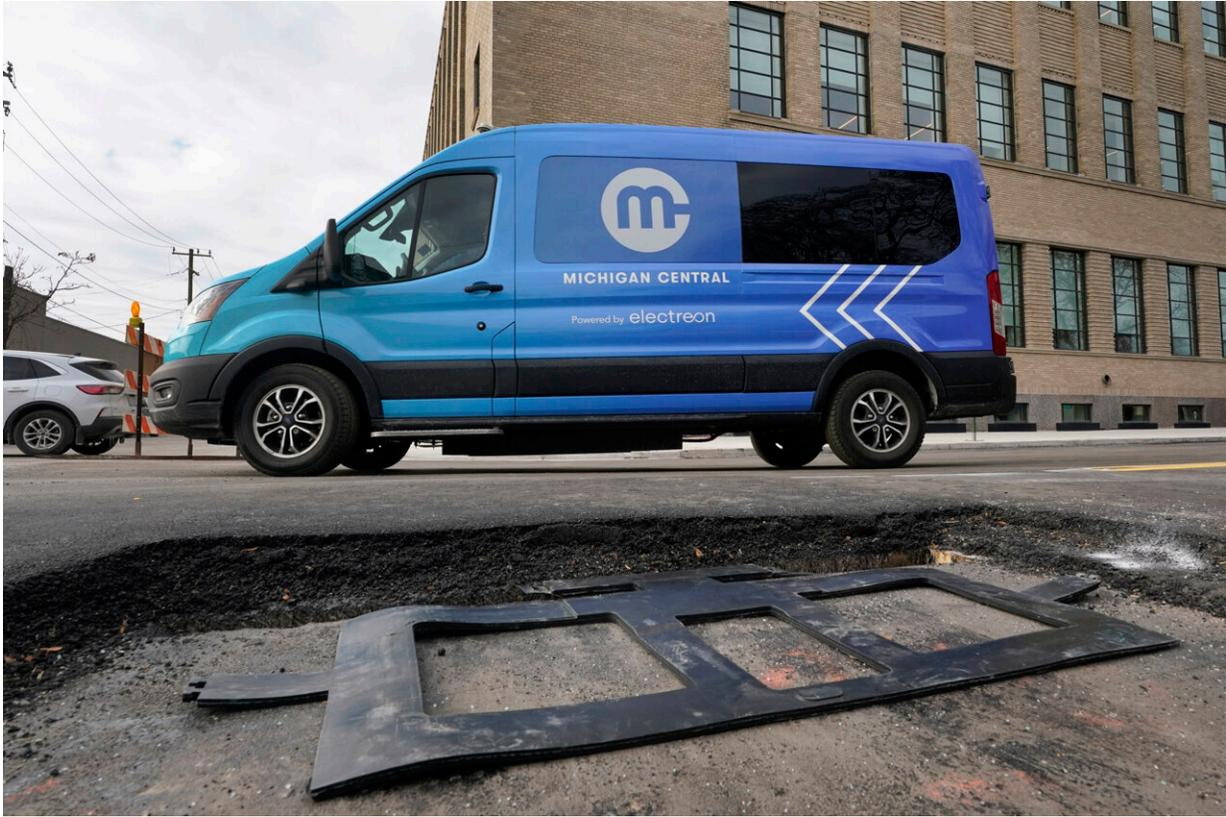
An electric van drives past a visible in-road wireless charging coil to be installed in a street in Detroit, Wednesday, Nov. 29, 2023. A demonstration of the first electric vehicle charging road in the U.S. took place Wednesday on a quarter-mile stretch of a Motor City street. Credit: AP Photo/Paul Sancya
