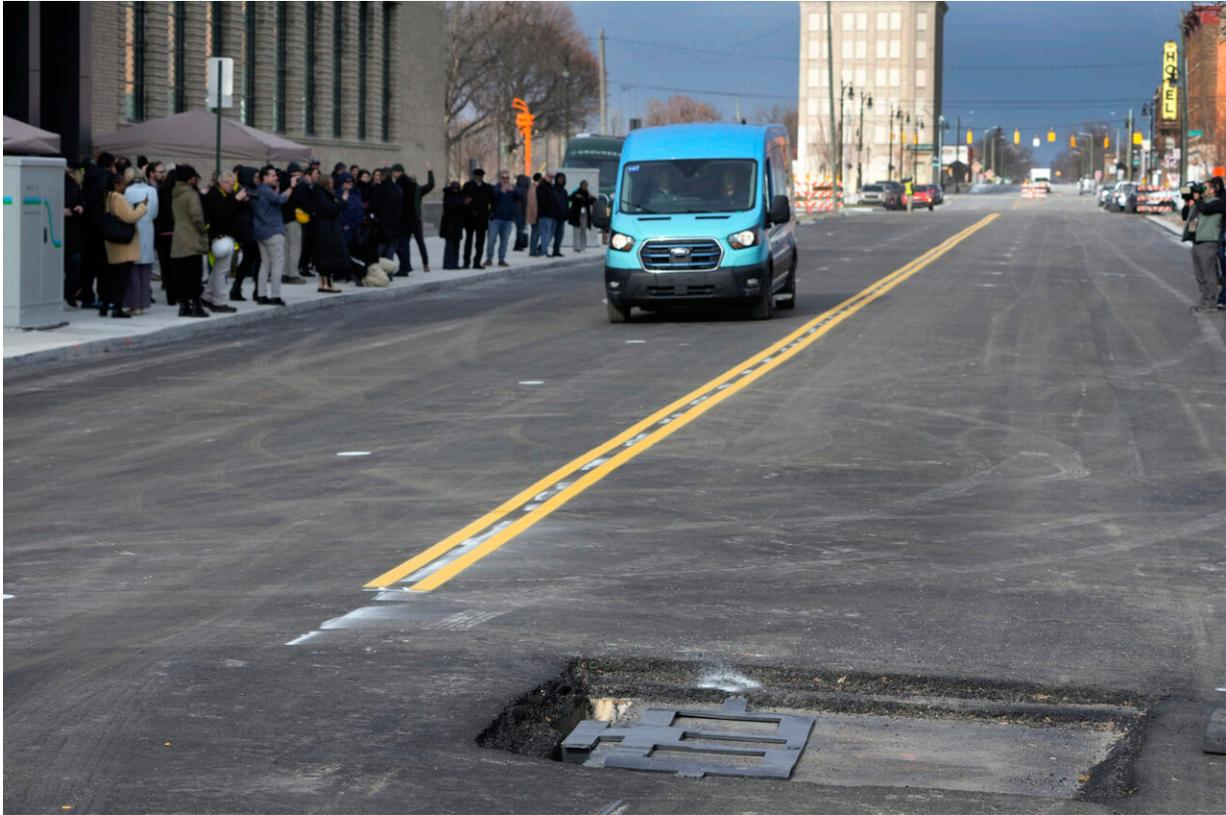
An electric van drives near a visible in-road wireless charging coil to be installed in a street in Detroit, Wednesday, Nov. 29, 2023. A demonstration of the first electric vehicle charging road in the U.S. took place Wednesday on a quarter-mile stretch of a Motor City street. Credit: AP Photo/Paul Sancya
