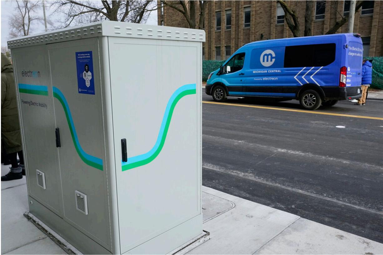
A management unit, left, which transfers power from the electricity grid to in-road wireless charging coil segments, is shown as an electric van drives down a street in Detroit, Wednesday, Nov. 29, 2023. A demonstration of the first electric vehicle charging road in the U.S. took place Wednesday on a quarter-mile stretch of a Motor City street. Credit: AP Photo/Paul Sancya
