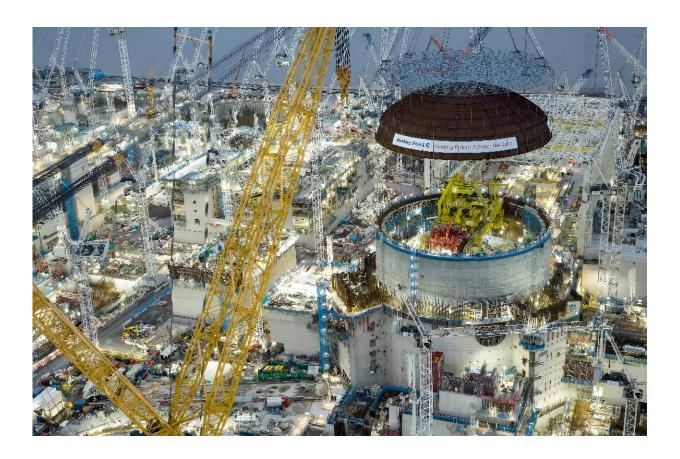
An EDF handout showing the steel dome being installed over Hinkley Point C's reactor 1.
