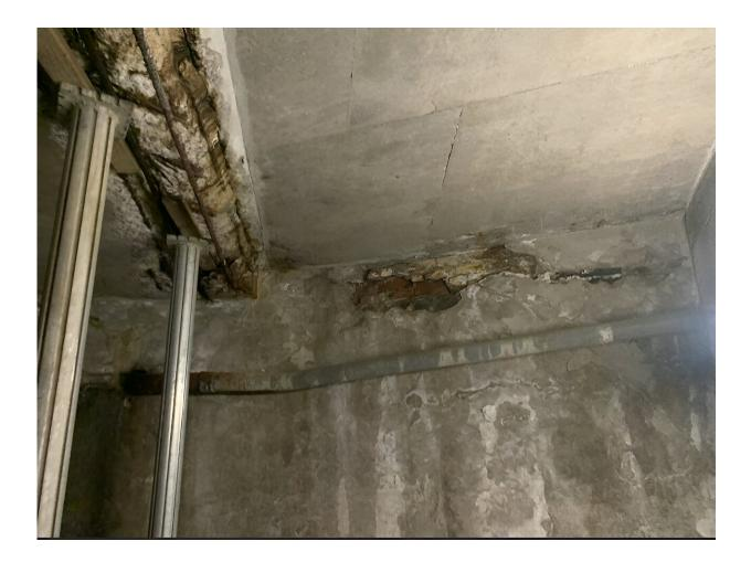
Deteriorating reinforced concrete and rusted or exposed reinforcing steel are warning signs to watch for. Credit: Jensen/BRV Engineering
