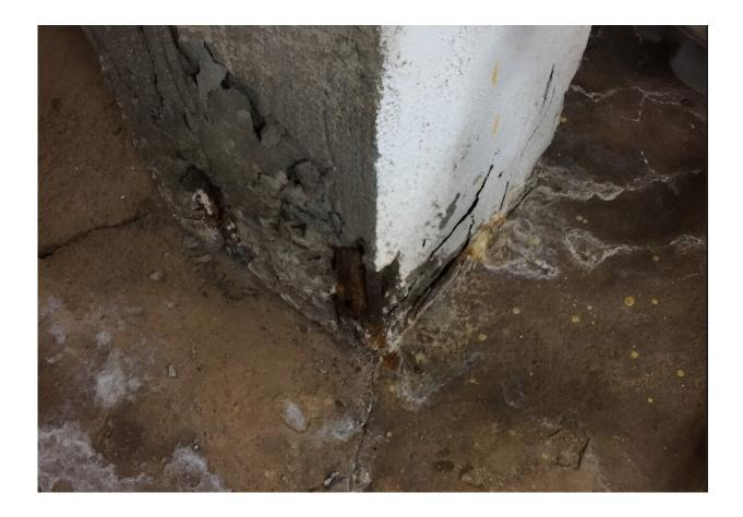
Signs of a degrading concrete column exposed to de-icing salt and moisture in a basement. Credit: Jensen/BRV Engineering
