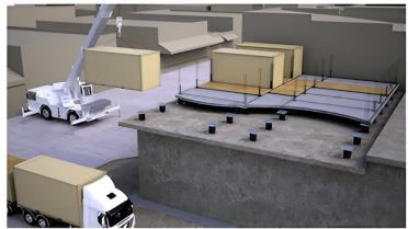
The components of modular housing are made in a factory and transported to the building site for assembly. Graphic illustration of modular construction methodology provided by UBC Smart Structures Lab, BC, Canada. Credit: Western Sydney University
