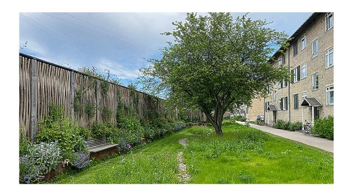
The breakthrough invention, disguised as a three-meter-high willow garden fence, is named the "Green Climate Screen." This solution has already been successfully implemented in the Copenhagen district of Valby. The Green Climate Screen doubles as a noise barrier and manages runoff from a neighboring building's roof, redirecting the water upward into the screen instead of sending it to a sewer. Credit: Department of Geosciences and Natural Resource Management.
