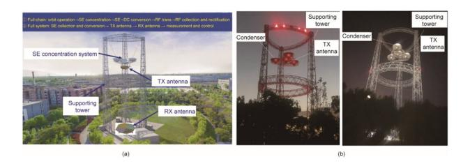
(a) Outdoor OMEGA-SSPS ground demonstration and verification system, and(b) prototype of OMEGA-SSPS ground demonstration and verification system.SE: sun energy; TX: transmission antenna; RX: receiving antenna. Credit:Baoyan Duan et al.
