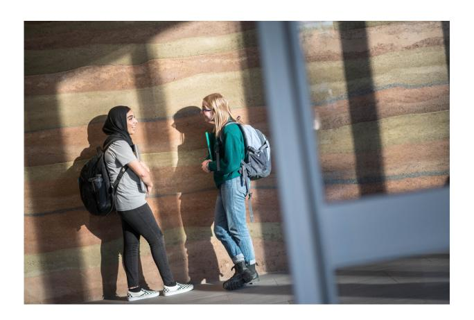
Rammed earth technology, where waste products such as fly ash, are used as sustainable building materials can also be used to make decorative feature walls like this one at UBC Okanagan. Credit: UBO photo
