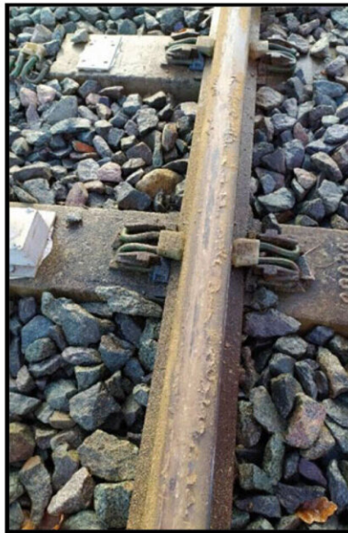
intermediate film (IMF) after rolling passes
