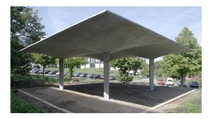
Picture from the construction of a pavilion at the RWTH Aachen University of Technology in Germany. The shell-shaped roof structure has been reinforced with carbon fiber textile and is only six centimeters thick. Credit: Robert Mehl
