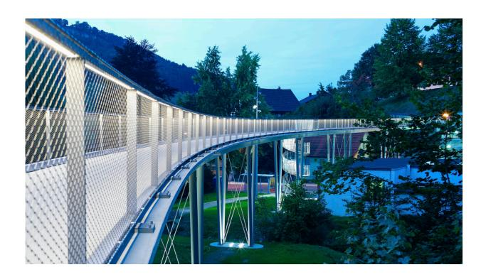
The pedestrian and bicycle bridge in Albstadt, Germany, is an early example of a textile-reinforced concrete structure. The bridge is about 100 meters long. Credit: Udo Jandrey
