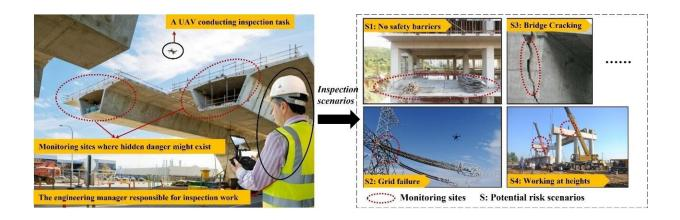
The UAV-based inspection approach has great advantages for performing inspection tasks in a complex and high-risk construction environment in order to continuously screen out potential hidden dangers. Credit: Lu Zhen, Zhiyuan Yang, Gilbert Laporte, Wen Yi, Tianyi Fan
