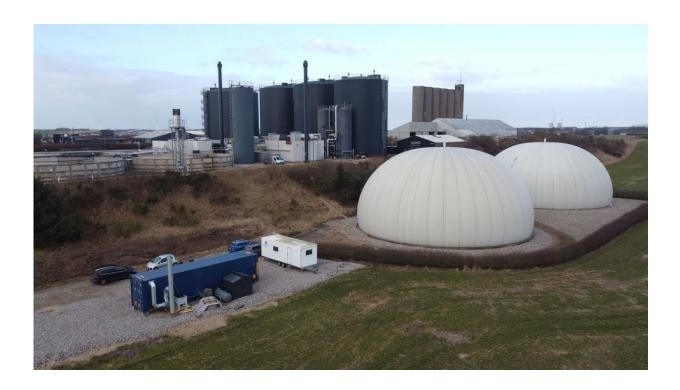
From Lemvig Biogas's large plant in the background, biogas is transported to the white domes and on to DTU's reactor in the blue container. Here the first green methanol has been produced. Credit: DTU
