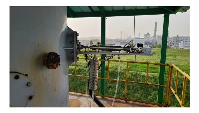
Equipment installed at a demonstration site (a waste incinerator in Korea) and carrying out continuous measurement. Credit: Korea Institute of Machinery and Materials (KIMM)
