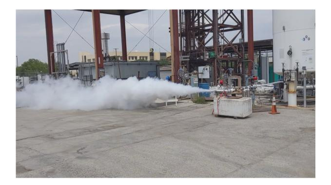
In this image, liquid nitrogen is expelled through a pressure relief valve as part of
