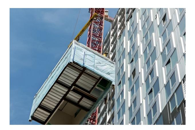
A living space module is hoisted in Brooklyn, New York, for installation into the world's tallest modular building. Natural-material floor cassettes could one day replace traditional steel-and-concrete surface assemblies in multistory buildings. Credit: SHoP Architects
