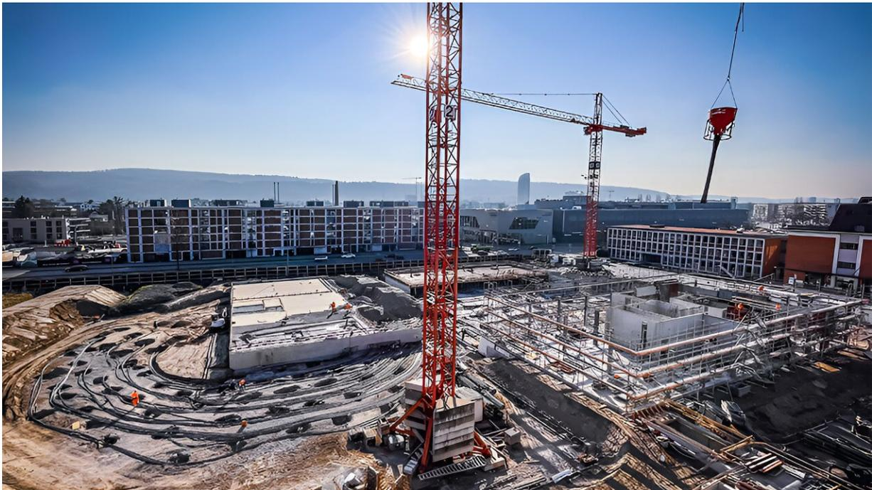
The new Empa campus in Dübendorf and the recently completed thermal energy storage field with 144 boreholes are a pilot plant in the EU GOES project. The aim of the project is to develop an initial application for platform-based design. Credit: Empa
