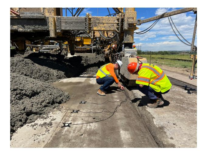
Purdue University researchers and the startup Wavelogix worked with a crew to test REBEL sensor technology, invented by Purdue, within a section of Interstate 25 in Colorado last summer. Credit: Purdue University /Rui He
