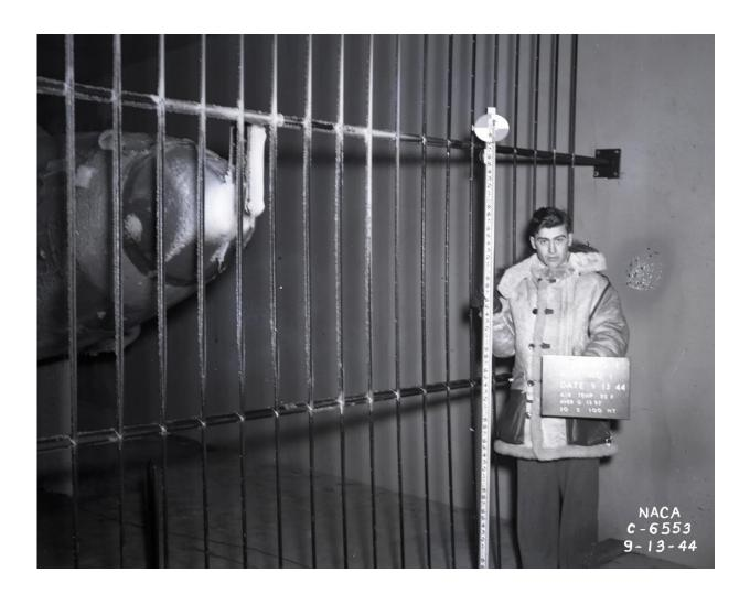
A National Advisory Committee for Aeronautics researcher notes the conditions on the P-39L after its first test run in the Icing Research Tunnel on Sept. 13, 1944. The aircraft was too large to fit in the test section, so it was installed downstream in a larger area of the tunnel. The initial tests analyzed ice buildup on the nose, propeller blades, and antennae. In the summer of 1945, the P-39L
