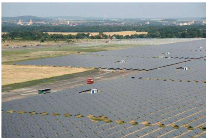
Solarkraftwerk Waldpolenz, the first Solar 40-MW CdTe PV Array installed by JUWI Group in Brandis, Germany. Credit: JUWI Group
