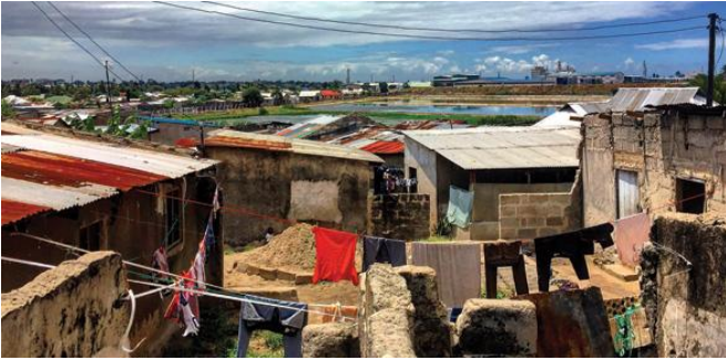
Dar Es Salaam. Credit: Izhan Khan
