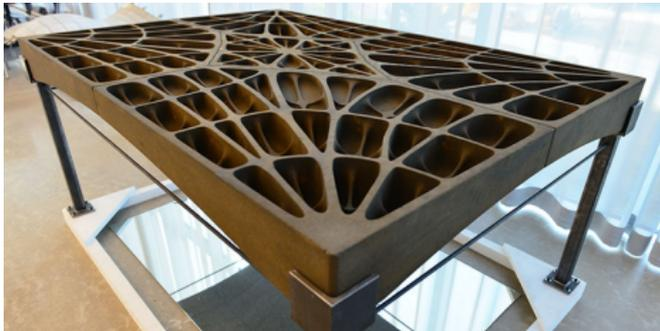
The construction of the unreinforced flooring, which is made up of individual slabs, takes its inspiration from Gothic cathedrals. Credit: Peter Rüegg / ETH Zurich
