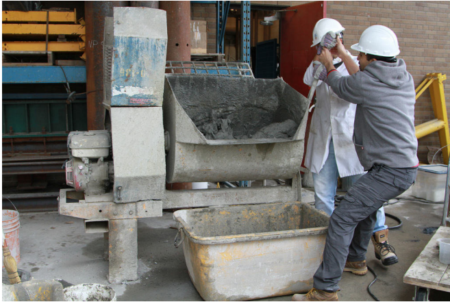
Mixing seismic-resistant concrete at UBC. Credit: UBC
