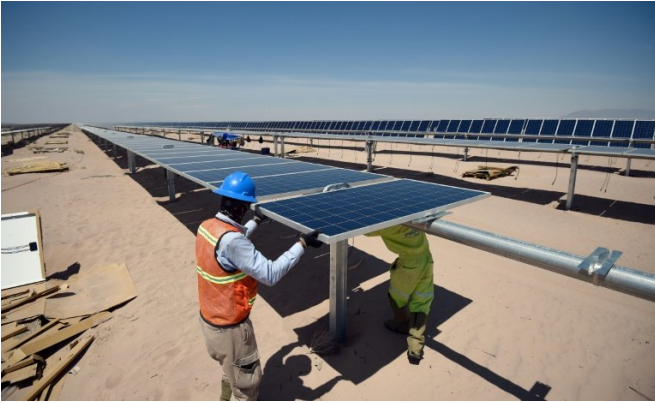
Workers install new solar panels at a power plant in the desert near Villanueva, Mexico, taken on April 20, 2018
