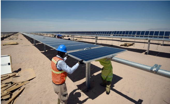
Workers install new solar panels at a power plant in the desert near Villanueva, Mexico, taken on April 20, 2018
