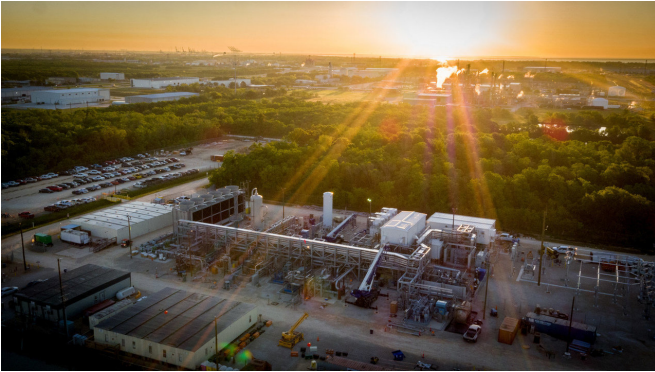
NET Power's 50 MWth Demonstration Plant in La Porte, Texas
