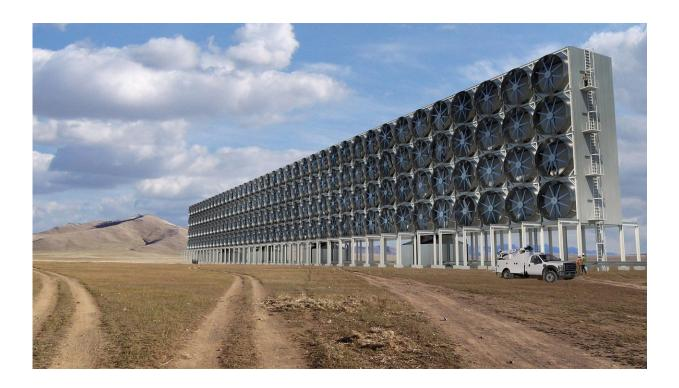
Artist's rendering of Carbon Engineering's air capture design. This unit would be one of several that would collectively capture 1 million metric tonnes of CO2 per year. Credit: Carbon Engineering
