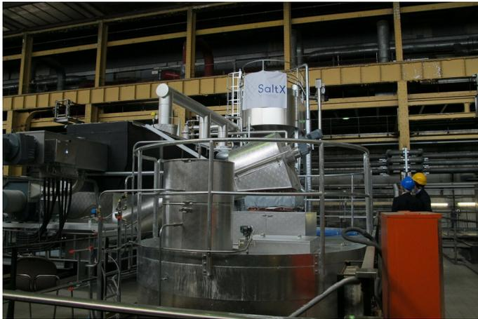
Personnel look up at an experimental salt-based heat storage facility at Berlin's Reuter thermal power station on Wednesday, April 24, 2019. The energy company, together with a Swedish start-up, is testing the use of salt to store heat, which accounts for more than half the power consumed in Germany. (AP Photos/Frank Jordans)
