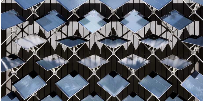
The movable solar panels harvest around 50 percent more energy than static solar panels. Credit: Arno Schlüter
