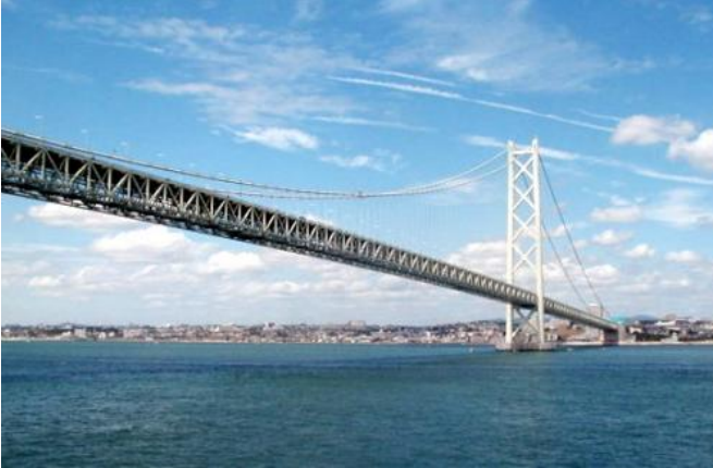
The Akashi-Kaikyo Bridge in Japan, the world's longest suspension span. Credit: Wikipedia
