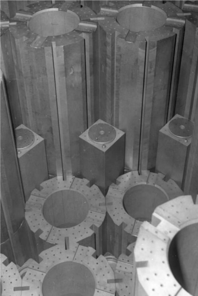
The structure of Graphite blocks in a nuclear reactor.
