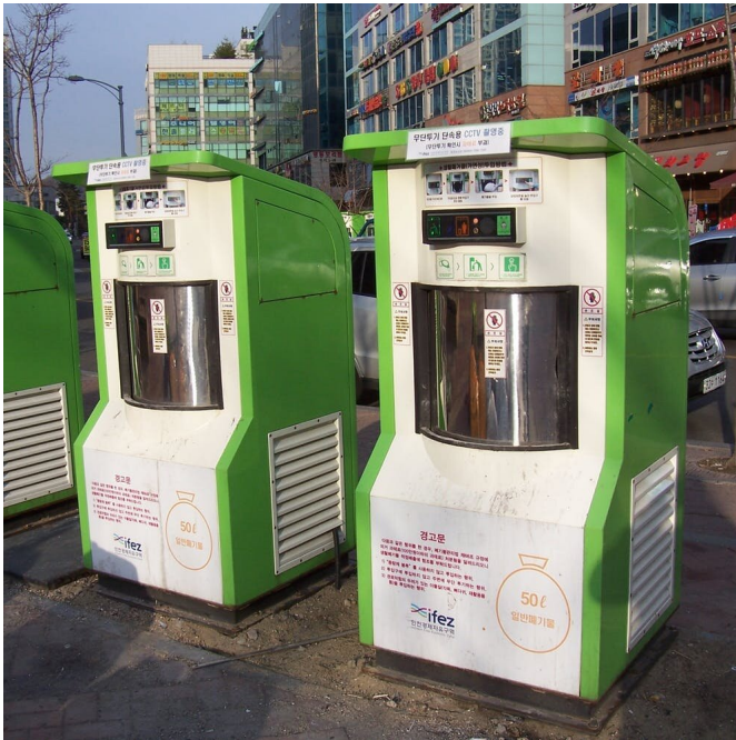
Automated waste disposal bins are connected via underground pipes to a waste-processing centre. Credit: Weli'mi'nakwan/Flickr, CC BY
