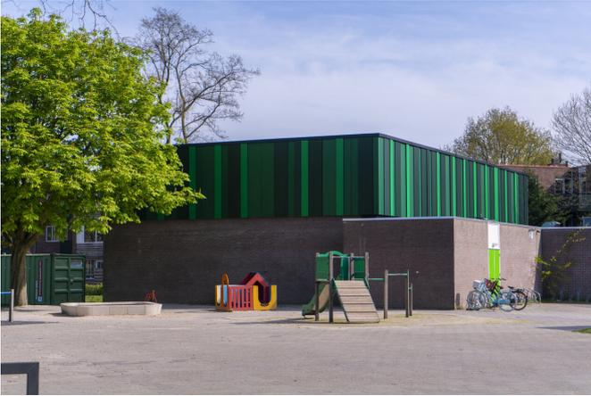
A coat of special green paint used on panels at a school gym in Almere, the Netherlands, helps the panels absorb sunlight for heating and for hot water. Credit: Emergo
