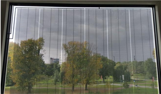
Photovoltaic windows contain embedded solar panels that can harvest electricity while still letting in light. Credit: TNO & NSG Pilkington
