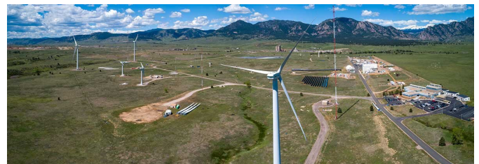
A hybrid power plant at NREL's Flatirons Campus, where grid-scale utility assets and numerous renewable energy and storage technologies come together for integrated energy systems research. Credit: National Renewable Energy Laboratory
